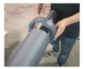
3. Put down section of solar cylindrical from top of pole(with cable position down forwards), go though cable of solar panel from pole(take off cable from solar cylindrical while go through solar cylindrical as below pictures:
