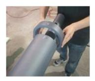
3. Put down section of solar cylindrical from top of pole(with cable position down forwards), go though cable of solar panel from pole(take off cable from solar cylindrical while go through solar cylindrical as below pictures:
