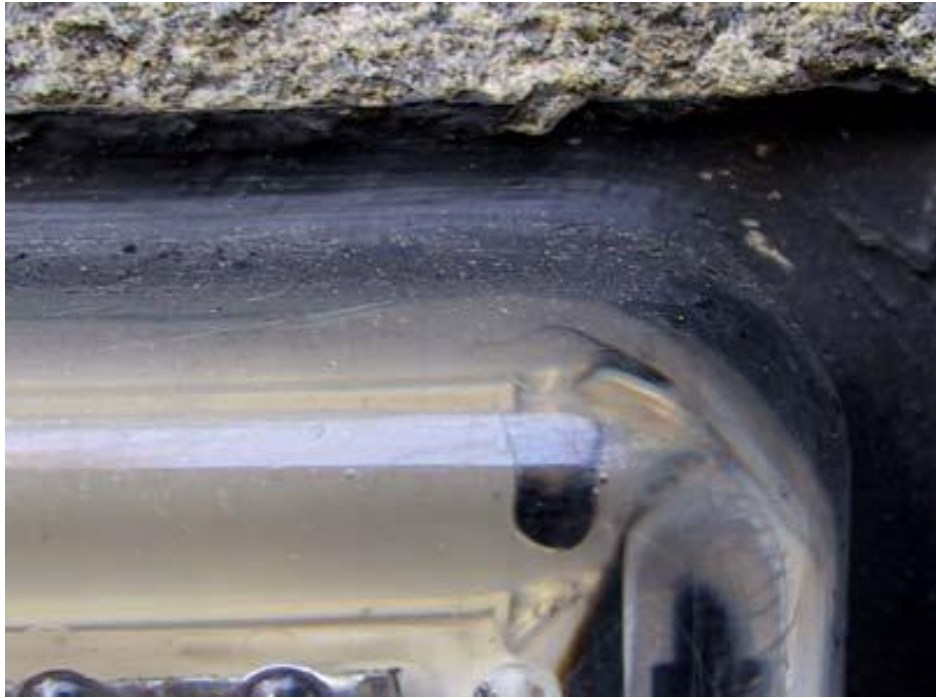
Installation using Silicone
