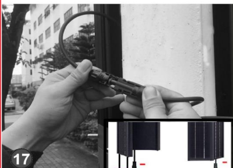
17 Connect the first module to the second module by MC4 plugs directly.
