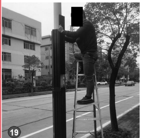
19 Put the second sub module on the bracket in the same way as 7 mentioned.
