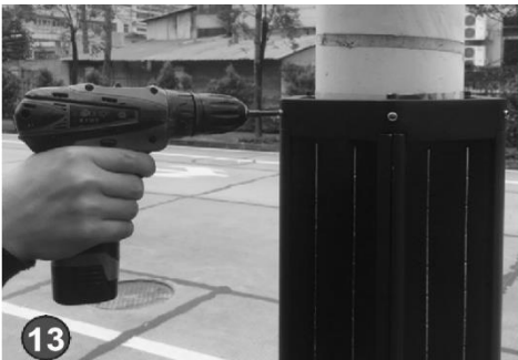
12 Adjust the position of the brackets at the best position. Similarly, let the pole in the middle of the hexagon brackets.
